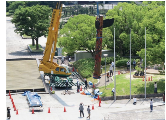
Photo 22 Erecting the totem pole (Photo by Mayumi Nishishita on June 24, 2020)
