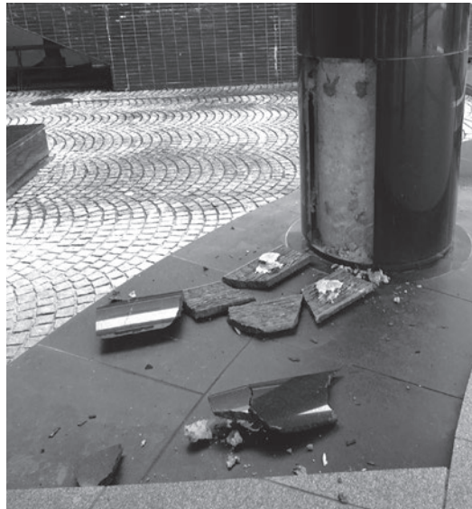
Exterior cladding that fell during the earthquake of June 18, 2018, at the public entrance to Minpaku.
