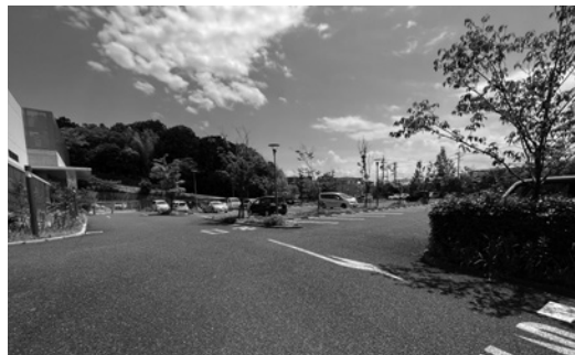
Heat exchange boreholes are buried under the parking lot of Mie Prefectural Museum (K. Suemori, 2022)
